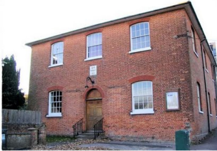
New Mill Baptist, near Tring, Hertfordshire
