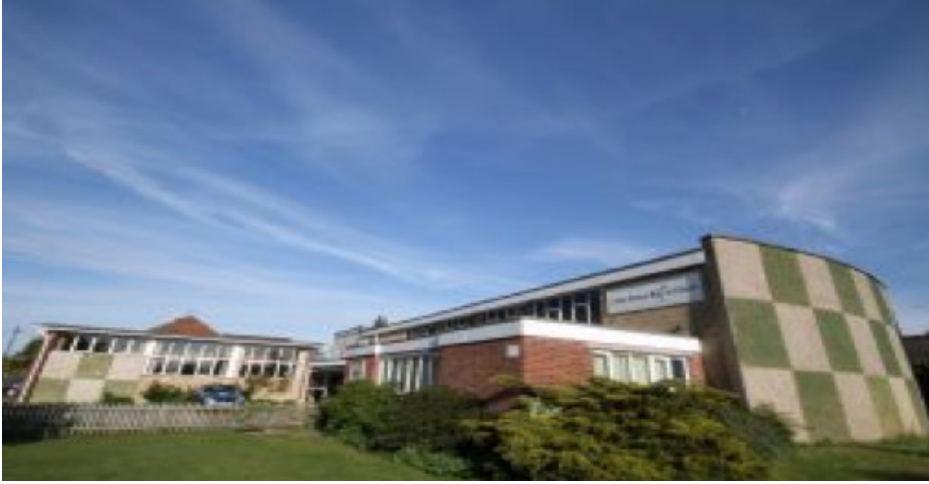
Limes Avenue Baptist Church, Bedgrove Estate Aylesbury.
