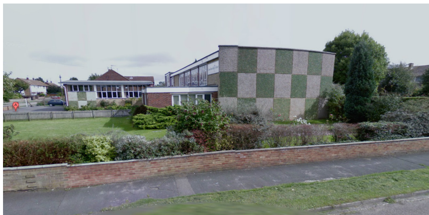
Limes Avenue Baptist Church, Bedgrove Estate Aylesbury.
