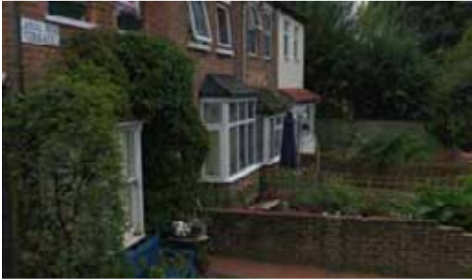
3 Canal Side Terrace, Aylesbury. My first House
