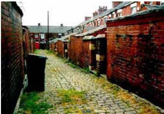
Back Alley at 26 Fleet Street
