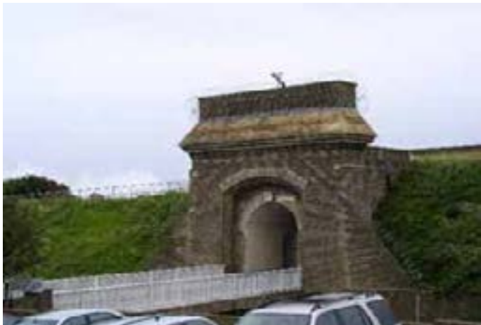
Dover Borstal (The Citadel)
