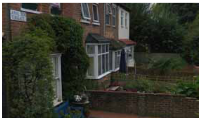
3 Canal Side Terrace, Aylesbury. My first House
