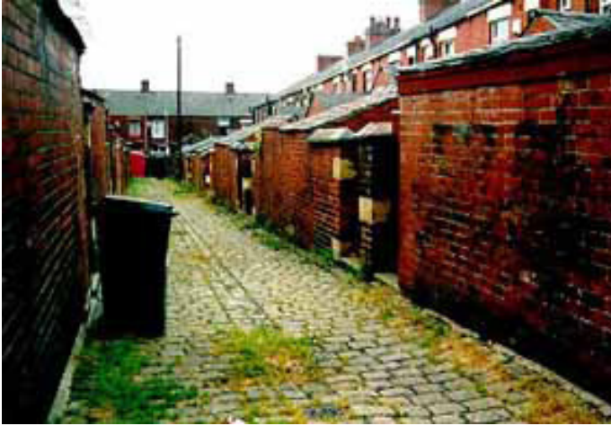
Back Alley at 26 Fleet Street
