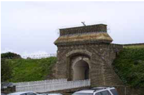
Dover Borstal (The Citadel)
