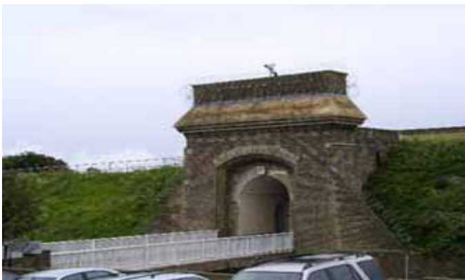
Dover Borstal (The Citadel)
