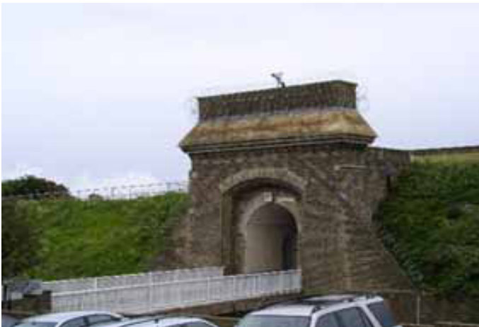
Dover Borstal (The Citadel)
