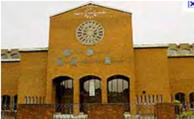
Martyrs Memorial Church building, Ravens Hill Road Belfast
