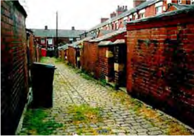
Back Alley at 26 Fleet Street
