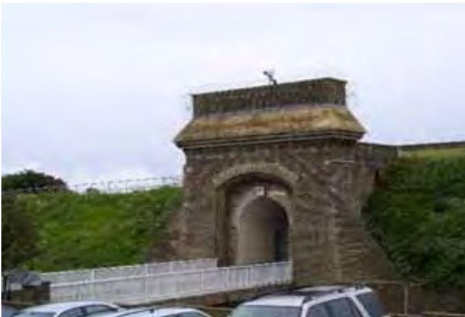
Dover Borstal (The Citadel)
