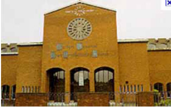
Martyrs Memorial Church building, Ravens hill Road Belfast
